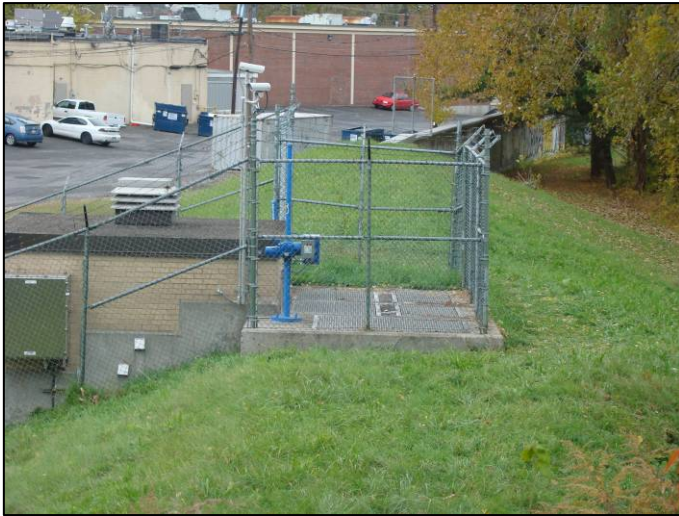
Figure 25: Army Corps of Engineers Levee behind Kingston Plaza from Col. Chandler Drive. This is the control gate to release water back to the Esopus if it collects behind the levee. - Photo by Gregg Swanzey
